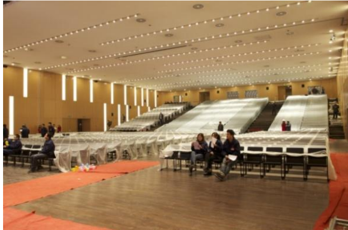
Figure 6 –Photo of the lecture hall (sand panels on ceilings)
